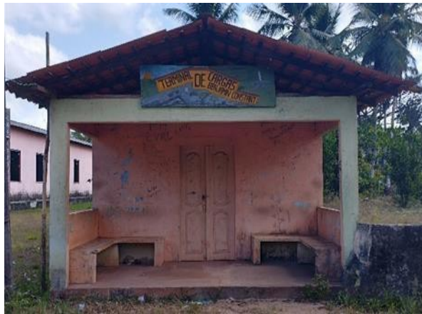
Figura 17: Antigo Terminal de Cargas Benjamin Constant
